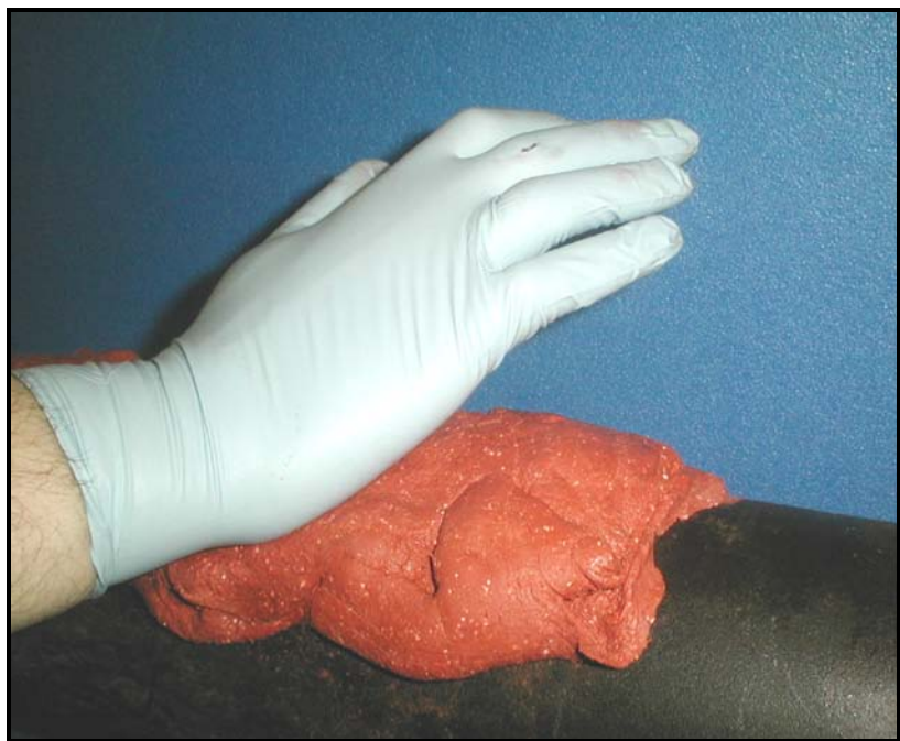
Figure 2-7: Applying DMP-3 Damping Material
